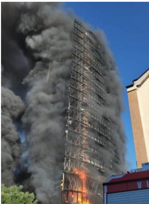
Figure 20: Most of the cladding has now been destroyed and the fire on the sail has burned itself out. However, the structural column (which extends behind the sail) continues to burn (left photo) and the interior of the flats (which the fire entered from the outside) are still alight.
