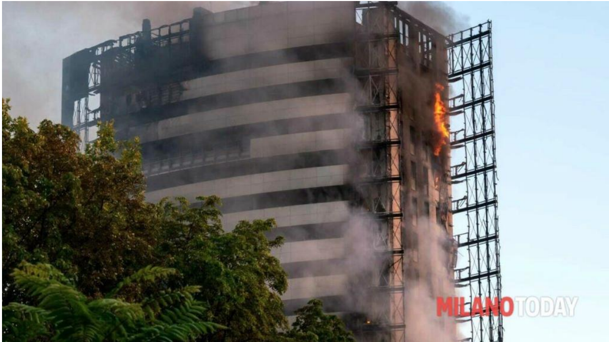
Figure 21: The tower viewed from the other side; the opposite one to where the fire started. The fire has spread around both ends of the building to affect both ends of the sail. On the left side there is evidence of horizontal fire spread along the balcony walls. There is also evidence of extensive fire spread via the perimeter of the roof.
