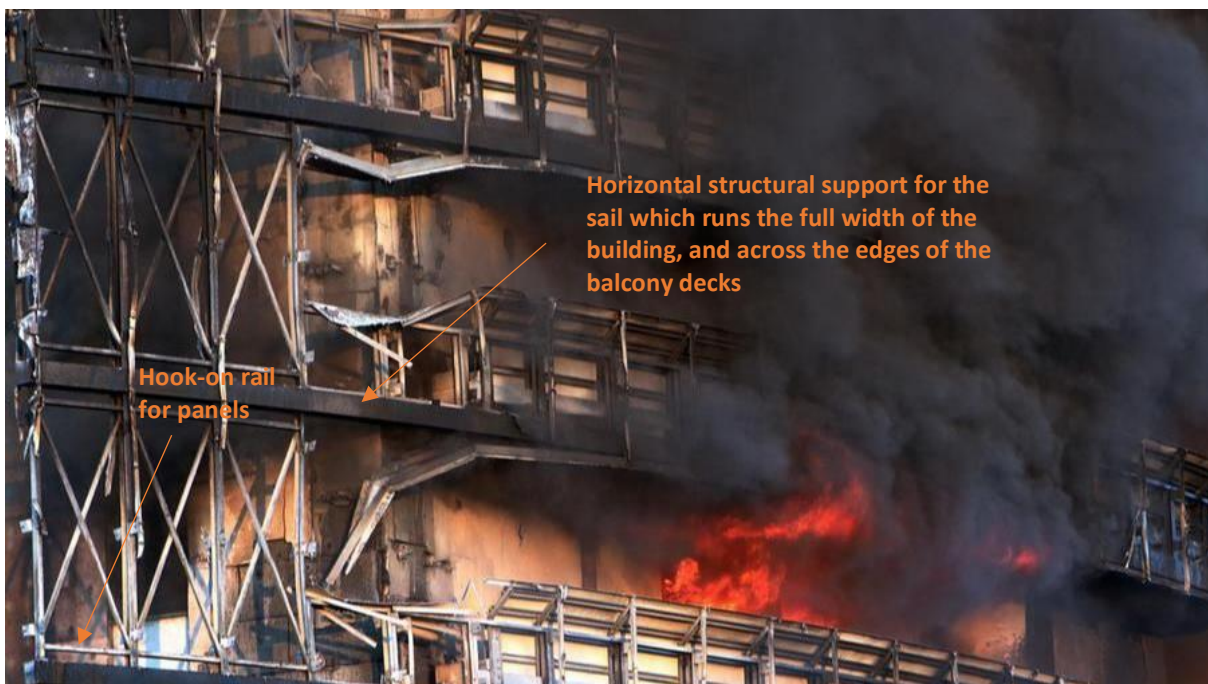
Figure 16: The same areas of the structure in Figure 15 above, but during the fire, where flames can be seen venting through the doors and windows of one of the flats.
