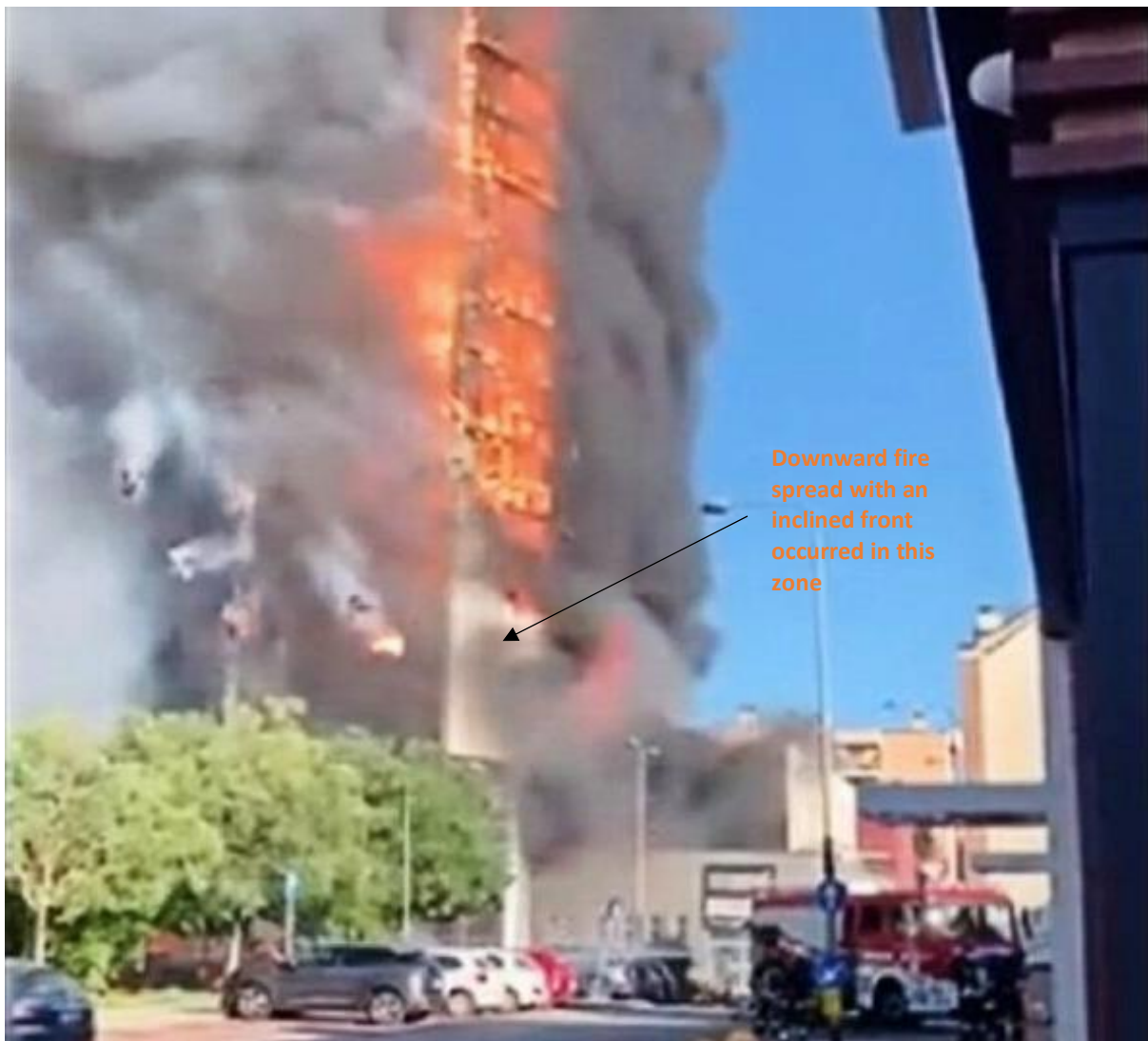
Figure 9: The fire started on the 15 th floor and spread across the building and downwards, as the cores of the panels melted and burned. In the lower corner of the building, just below the main band of fire and the tree tops, a diagonal pattern can be seen. This is a still image taken from a video where it is easier to observe the effect in motion, although in both cases the large amount of smoke makes it difficult to see.
