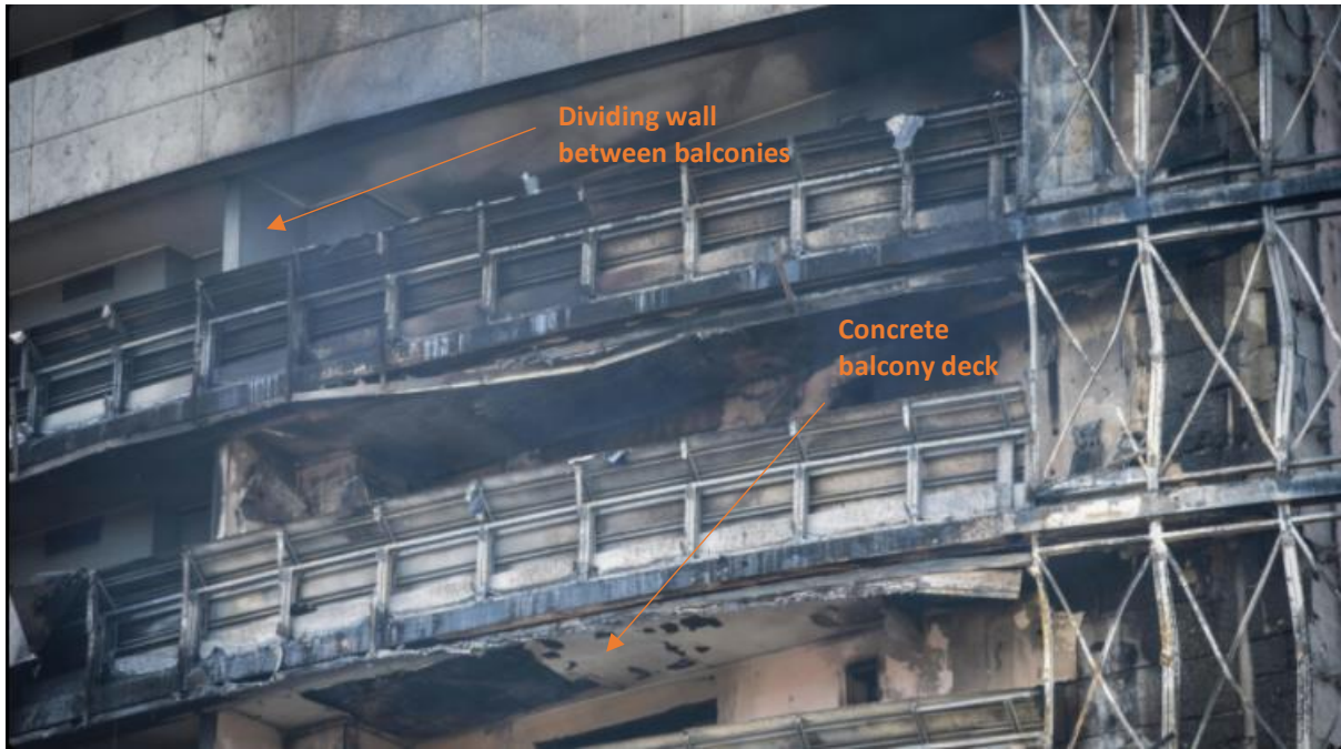
Figure 15: A close-up view of the balconies which shows the difference in the design of the framework with that on the ends of the sails. It is difficult to tell what lies behind the framework on the balconies, but whatever the material is, it has remained intact. The ends of the sails have burned through completely and the wall behind, at the interface with the core and the balconies, is exposed.
