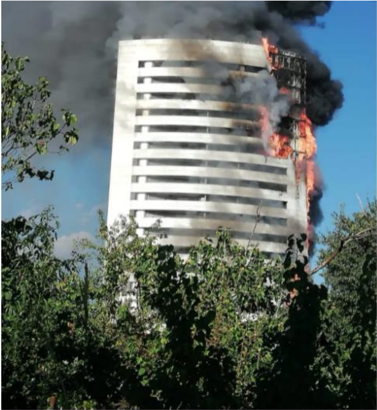
Figure 18: The fire is now well developed and has destroyed the cladding on the top right corner of the sail. It has spread upwards, downwards and horizontally from the flat where it started. It is now affecting the combustible material at the top of the sail, around the edge of the roof.
