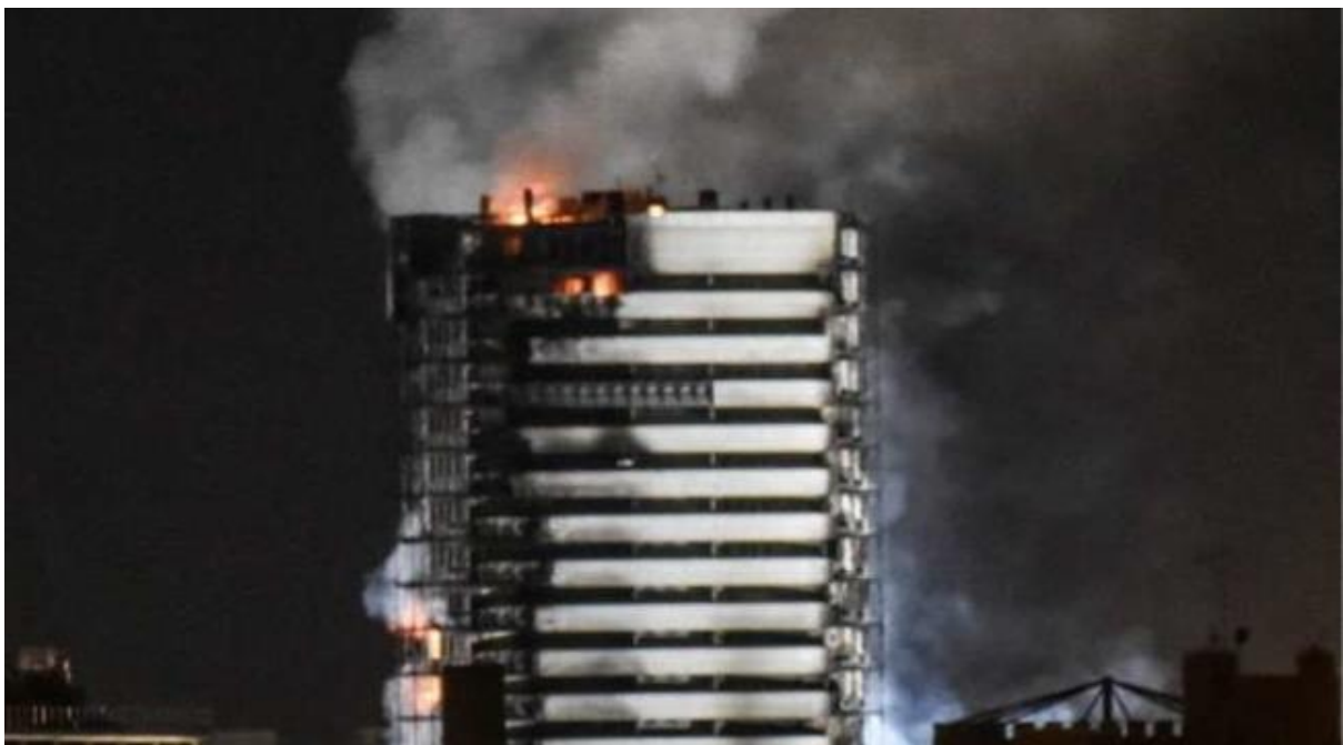
Figure 22: The same side is viewed again from a different angle, where flaming can be seen at roof level against the darkened sky.
