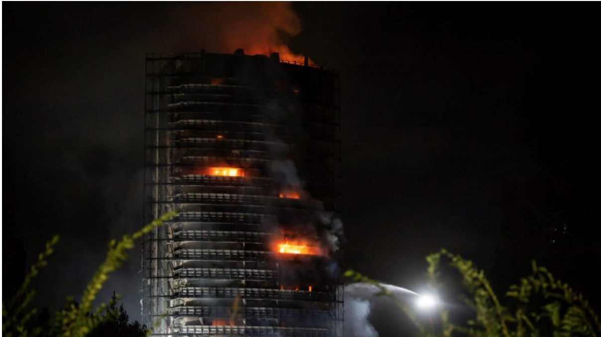
Figure 23: A night-time view of the side where the fire started showing that the interior of flats remain alight and there is still substantial flaming at roof level.
