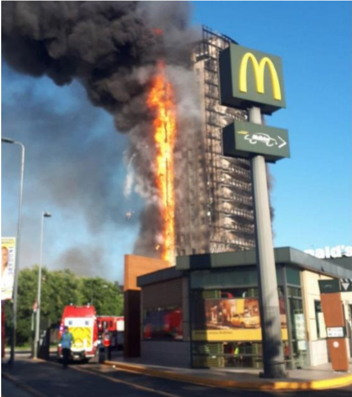
Figure 4: In this photograph the flames are concentrated within the vertex created at the interface where the sail projects beyond the edge of the core. The fire, having rapidly consumed the cladding on the sail, entered the corner where it became concentrated on a band of cladding.
