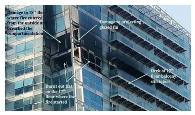
Figure 6: The Relay Building after the fire has been extinguished, where there is damage to both the 17<sup>th</sup> and 18<sup>th</sup> floors.
