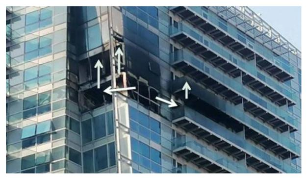
Figure 7: This is a repeat of *Figure 6*, but with the purpose of showing the various paths the fire took as it spread through the curtain walling system.
