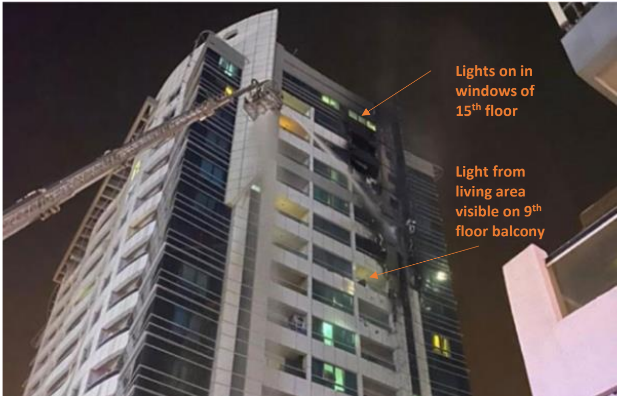
Figure 20: Most of the fire has now been extinguished and the firefighters are damping down. A light can be seen in the 9 th floor balcony, which is coming from the living area and projecting through the glazing of the balcony doors. It has illuminated the ceiling of the balcony which appears to be undamaged. The lights are also on in the 15 th floor flat where the damage is confined only to the external cladding. Photo: www.gulftoday.ae
