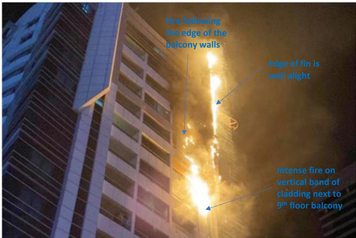
Marina Diamond 2 building on fire in Dubai.
