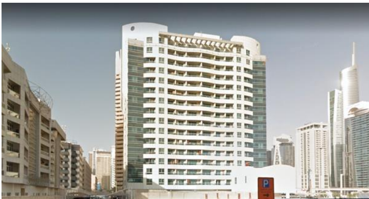
Figure 3: The south-west side of Marina Diamond 2 showing the curved corners which are covered in combustibile cladding. Glazed living areas protrude from these corners at right angles. The rest of the façade has a rippled effect, like waves in the sea. Photo: The Author
