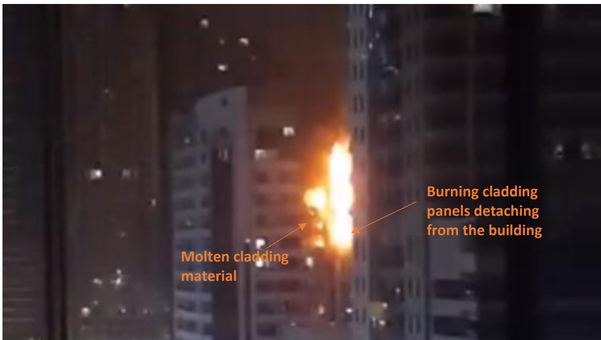
Figure 9: The upper floors on one side of the north-west of the Marina Diamond 2 are engulfed in flames, which can be seen spreading downwards as the cores of the cladding panels melt, flow and drip.
