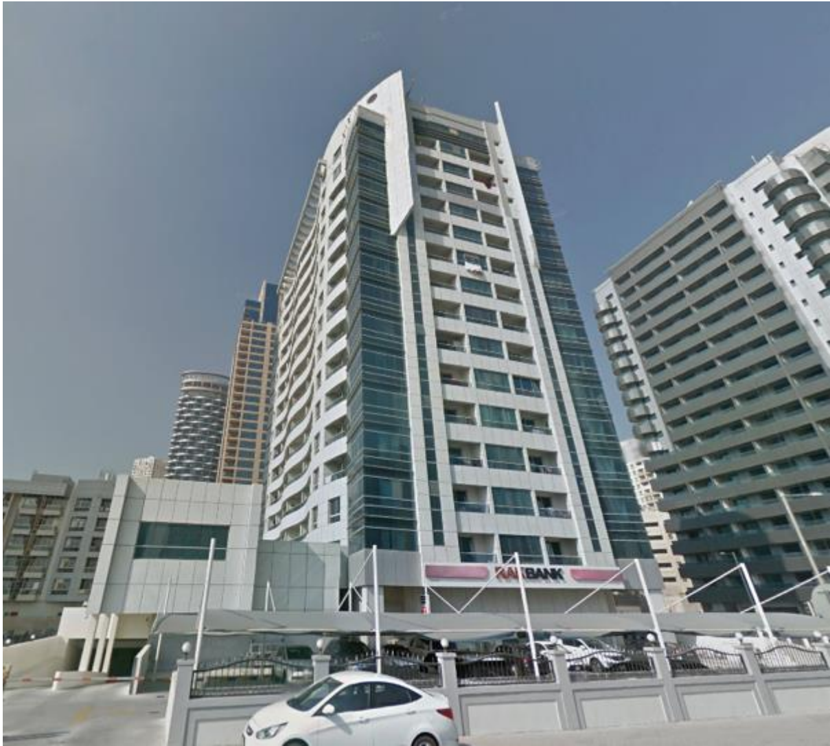
Figure 4: The south-east end of the building showing the fins which project beyond the curved corners from the tenth floor upwards. The fire occurred affected the opposite end of the building which is a mirror image of this one (see cover photo). Photo: The Author
