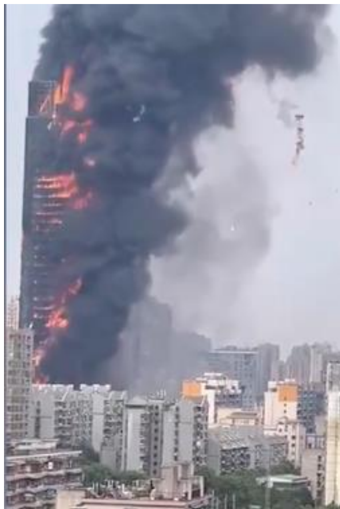
Figure 9: The fire can be seen here at a well-developed stage where it is affecting all levels on this side of the building. A diagonal front moves across the central curved section and flaming debris falls from the smoke cloud. The fire is following the line of the window cills and has caused the windows to fail at multiple levels.
