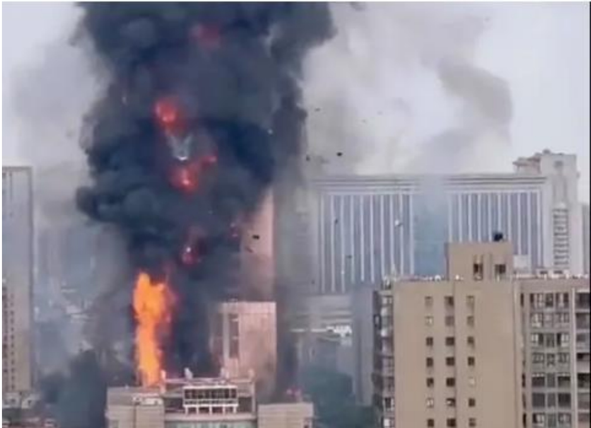
Figure 7: The fire began at the top of the podium on the left side of the building face as shown here. The cladding panels burned fiercely, producing a thick cloud of black smoke as the fire spread rapidly upwards and then across the building towards the other corner before it was finally extinguished. Many of the panels detached from the building as they burned and debris can be seen falling downwards.
