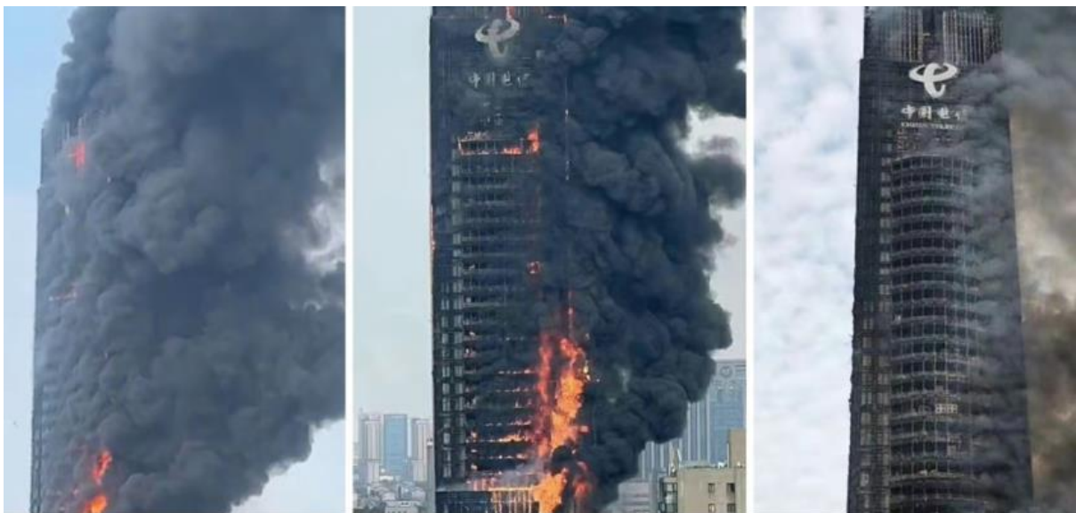
Figure 8: The photo on the left shows the fire at mid-stage of its development where the Coanda effect is also visible, which causes hot gases and smoke to be drawn back against the building face, as was also seen at
