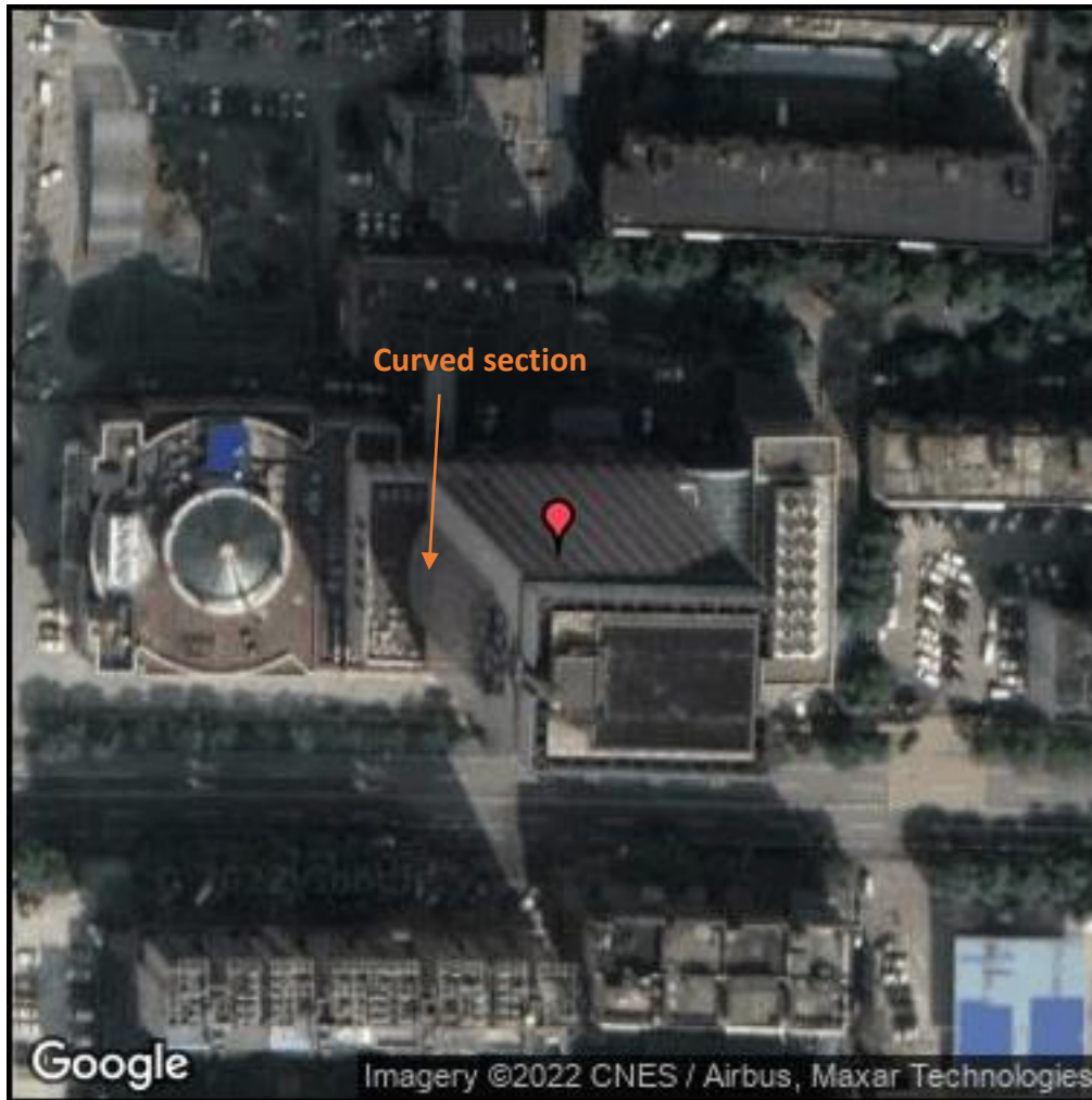
Figure 2: A Google image showing the tower from above and giving a good view of its geometric profile which had a profound influence on the way in which the fire spread and behaved. Of particular note is the curved section on the front elevation of the building which forms a vertex at the points where it joins with the main building face.
