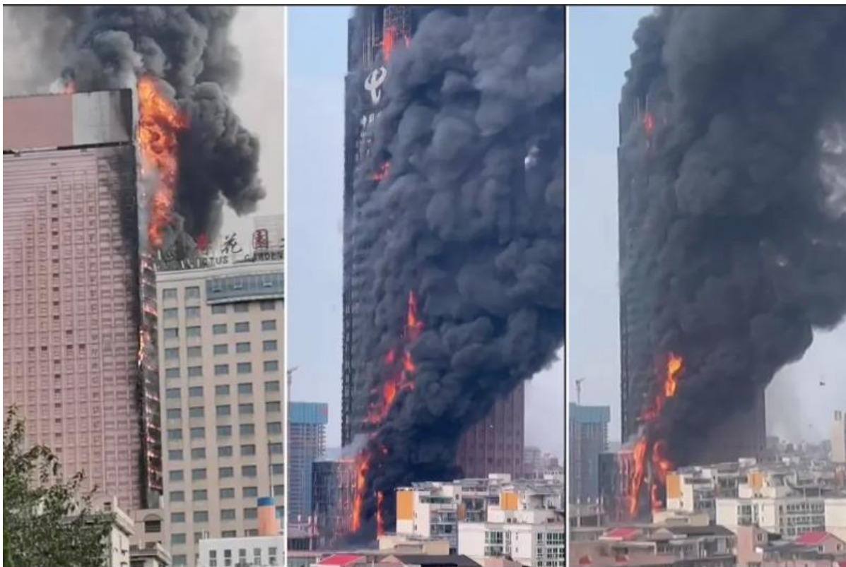
Figure 5: A series of three photos which show the fire at different stages of its development. The photo on the left shows a view of the building from the side, and apart from a slight blackening of the pinkish coloured cladding panels due to sooty deposits from the smoke, the fire has not been able to progress around the corner. The middle photo along with one on the right, show the podium on fire at lower levels with a column of flame spreading vertically upwards. The fire is also affecting the curved section in the middle of the tower and the front is diagonally inclined due to a differentiation in speed between the upper end of the fire front and the lower end of the fire front as the flames follow the line of curvature. The more pronounced the curve is, the greater the angle of inclination will be.
